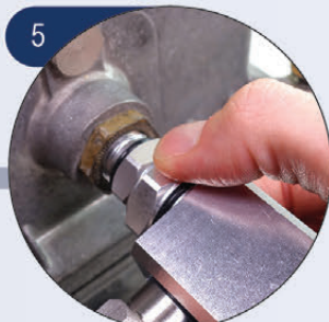
5 Thread coupling fitting into node (due to left-handed threading, coupler will thread simultaneously)
