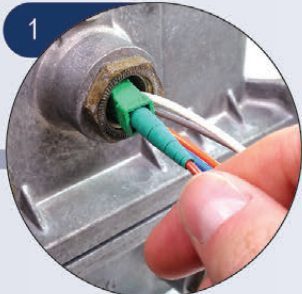
1 Feed connectors through node entry port
