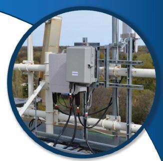
Amphenol's Fiber box is designed to be the easiest and fastest to install box solution on the market. The box is delivered preassembled, ready to connect to the fiber trunk and to any RRH with fiber optic jumpers.
