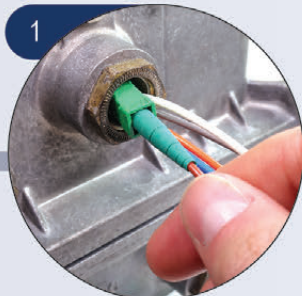
1 Feed connectors through node entry port
