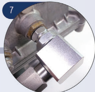
7 Field installation complete
