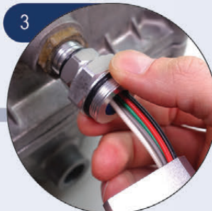
3 Thread coupling fitting a full turn into node
